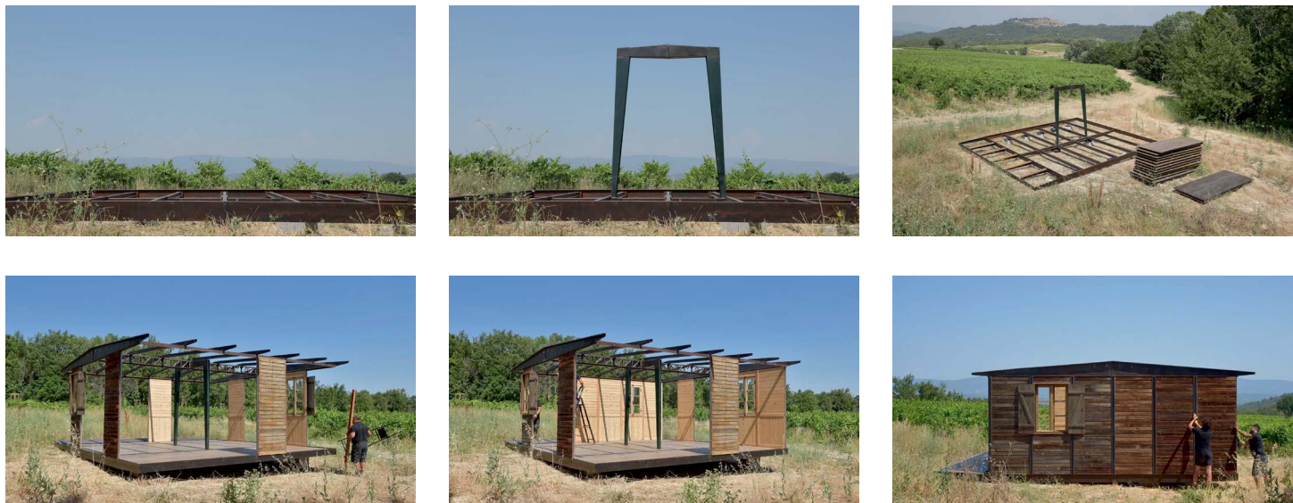
The 6 x 6 Demountable House at various stages of assembly
